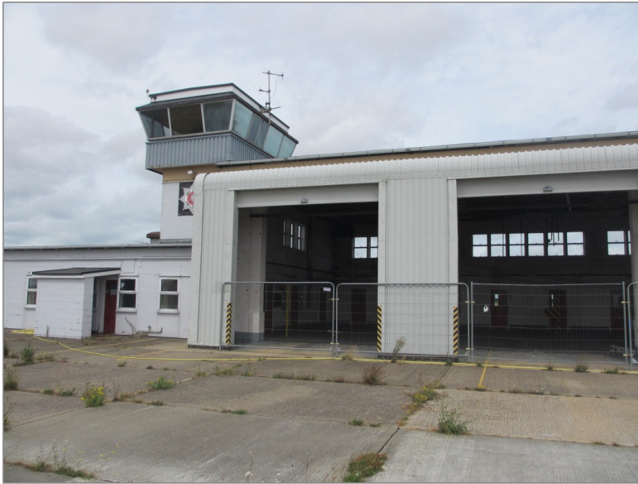
Figure 13: Dilapidated Rescue & Fire Fighting Facility
