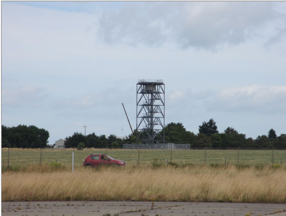
Figure 12: Radar tower with radar removed
