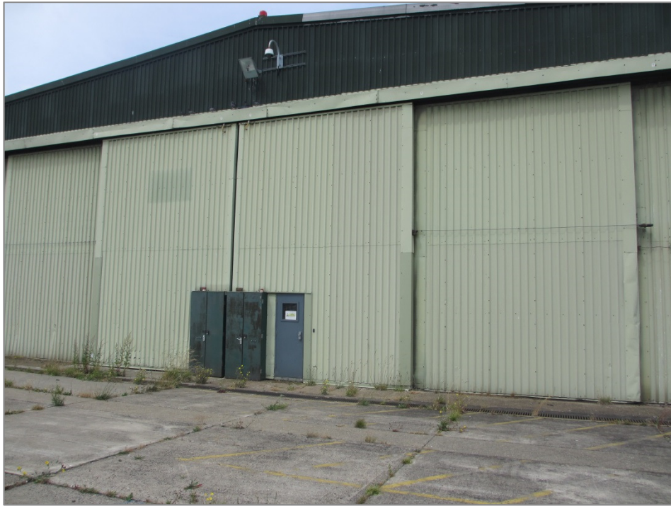
Figure 17: First cargo hangar exterior
